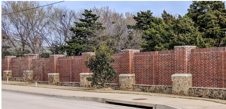
Figure 4.07.1. Example of Solid Masonry Wall
