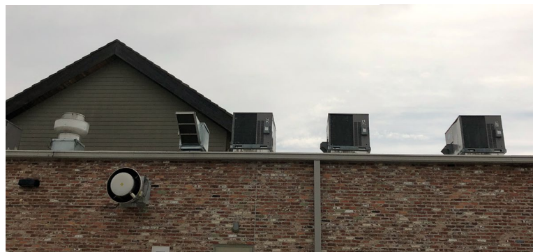
Figure 4.07.4. Example of Unscreened Rooftop
