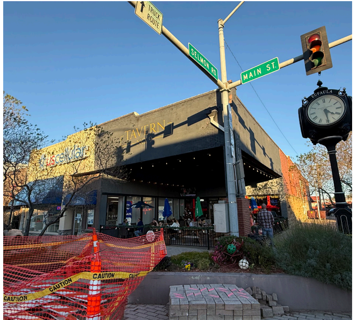
Construction at a Multimodal Intersection
