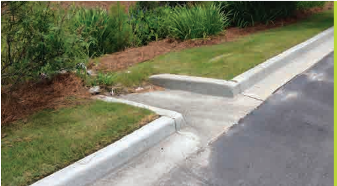
Example of Parking Lot Bioswale
