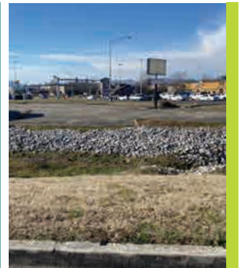
Existing Drainage Infrastructure
