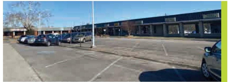
Existing Grove Center Shopping Center Parking Lot
